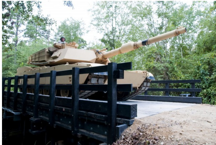
Figure 3.8 – Fort Bragg plastic bridge, taken the 25.09.2009 by Dawn Elizabeth Pandoliano [31]
